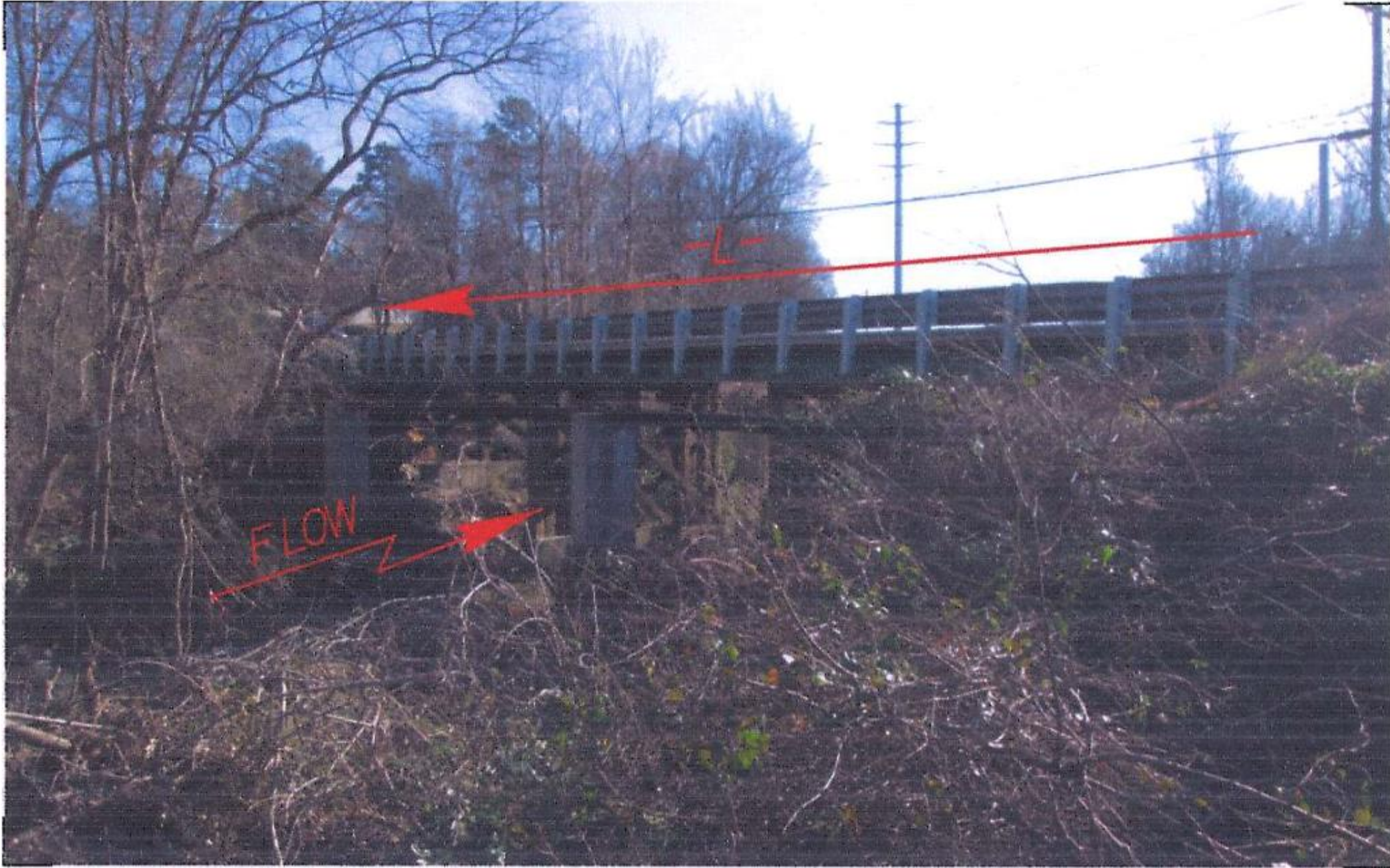
Looking South towards End Bent 2
